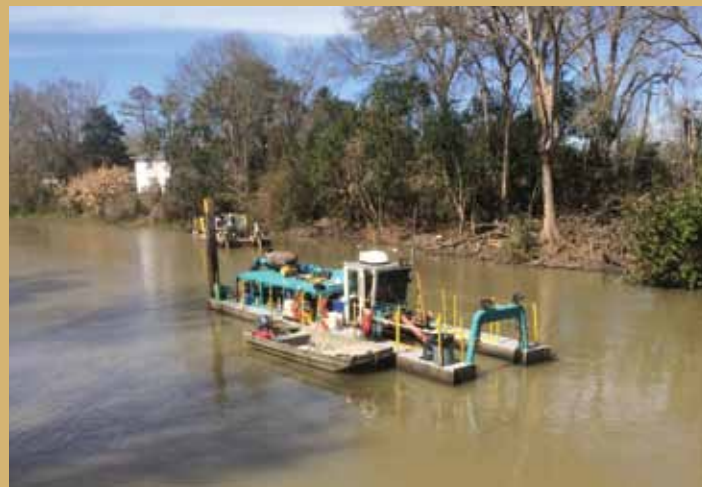
Bertucci dredge working in Bayou Lafourche.
